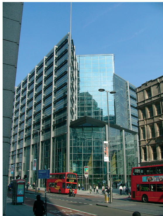
Left: ABN Amro – 300kW CO 2 mission critical cooling
